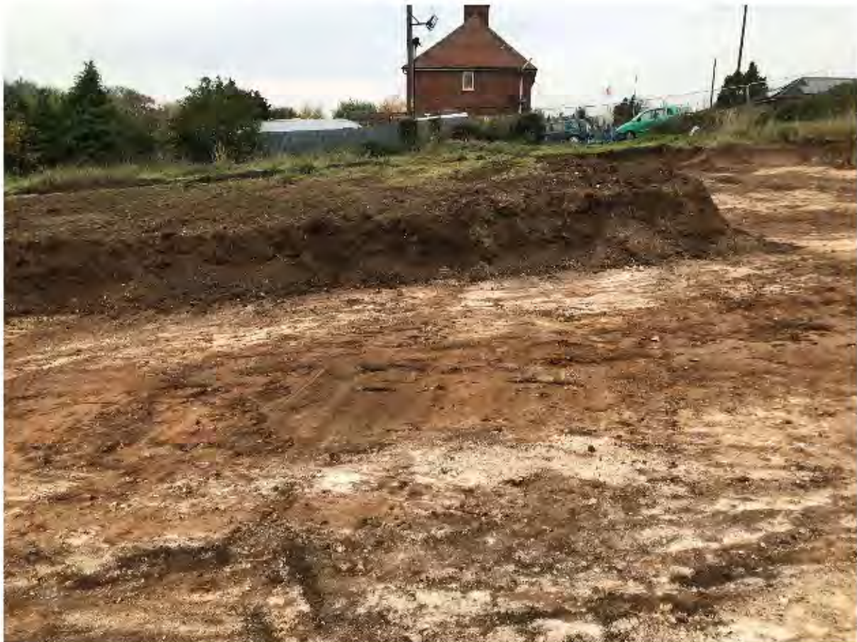
Image 25. Excavation down to solid chalk.
