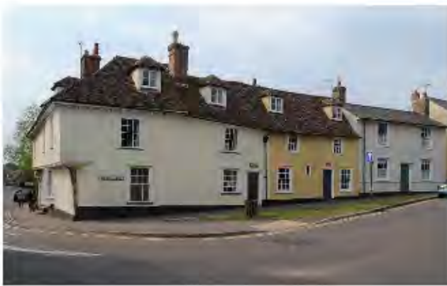
Image 11e. Grandest merchant houses in CA (the exception). Horizontal proportions, well-spaced openings. High quality natural materials, handmade clay tiles Roof pitches suit the vernacular materials.
